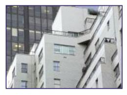
Above: 60 West 57th Street AM&G completely demolished and reconstructed parapets throughout the building, replacing corroding iron railings with aluminum railings.
